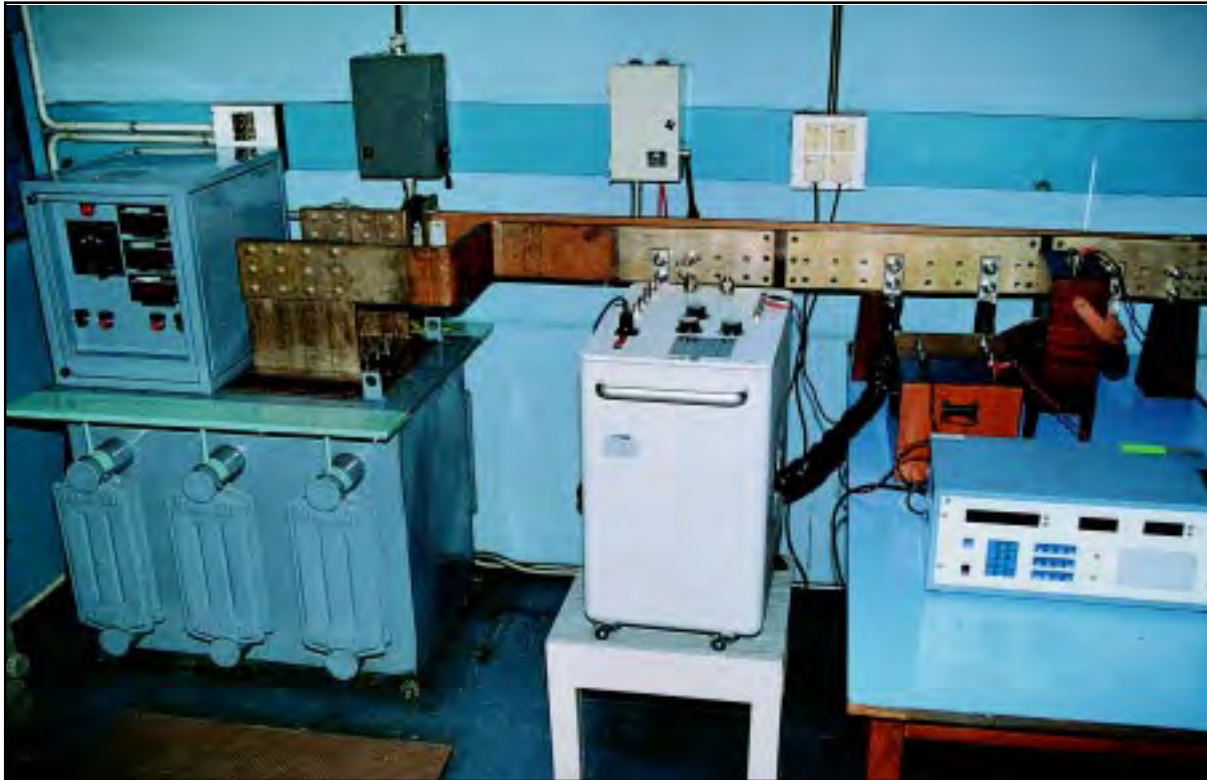
Fig. 2.6 : Experimental set-up for calibration of AC High Current Ratio (5A-5000A/1A,5A) at 50 Hz.
