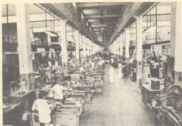
Fig.18: General view of the Workshop
